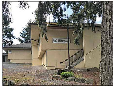
DRIFTWOOD FILE PHOTO Salt Spring Island Middle School, which will be fully closed for school use by next summer. The school district and Capital Regional District have approved in principle a five-year lease agreement that would see the building used as a community centre under CRD administration.
