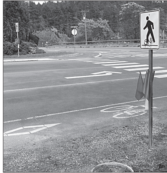
PHOTOS COURTESY SSI TRANSPORTATION COMMISSION SAFE AND SEEN: From left, Jon Scott tries out the new red flag safety system in place at the Lower and Upper Ganges Road crosswalk. Flags are also available at the McPhillips Avenue and Lower Ganges Road intersection, with additional installations coming at the Hereford Avenue and Lower Ganges Road crosswalk and the one on Lower Ganges Road near Village Terrace. Salt Spring Island Transportation Commission member Peter Meyer instigated and organized the project to help make pedestrian use of Ganges crosswalks safer.
