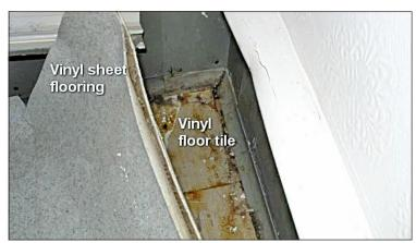
Two of several places where asbestos can be found in homes built before 1990 in B.C.: in the attic and in vinyl floor tiles and sheets.
