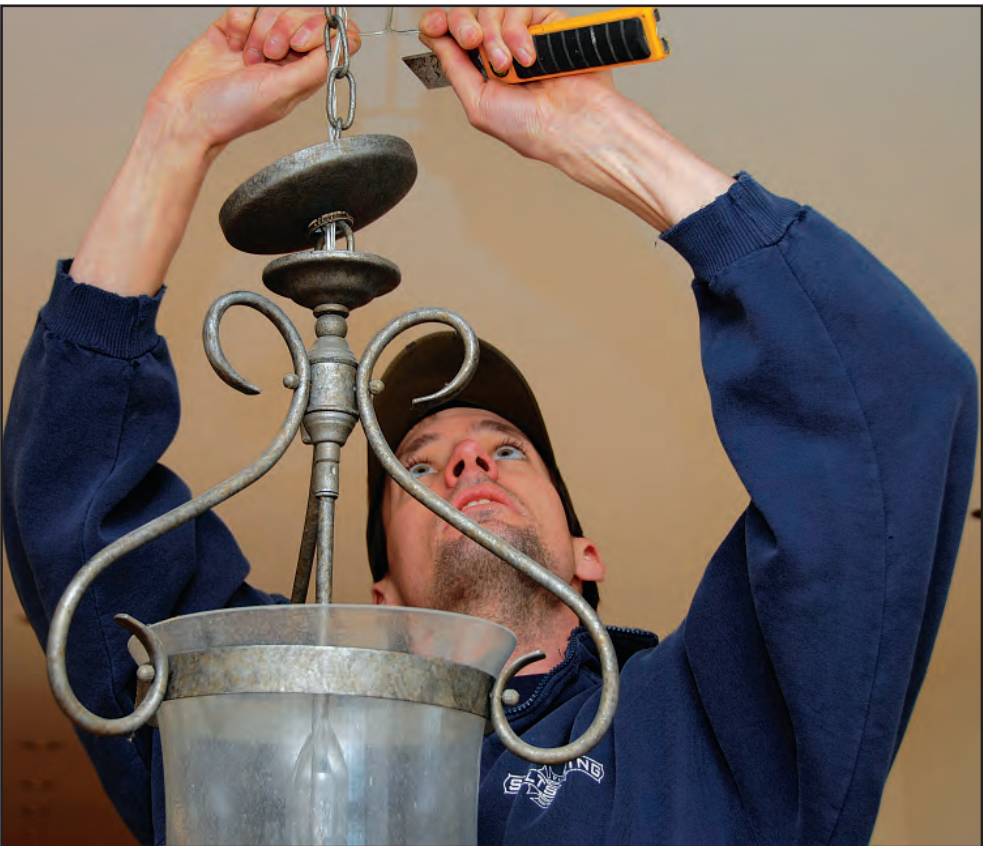
HOME MAKEOVER: Ken Akerman checks the circuit before installing a hanging lamp at a home on Salt Spring. Photo by Derrick Lundy
