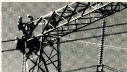
500 KV line repair near Whistler.
