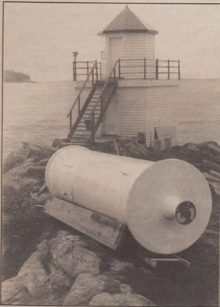
LIGHTHOUSES OLD AND NEW: New fiberglass tower, like the one in foreground, will replace the wooden one behind it as lighthouse automation begins in B.C.
