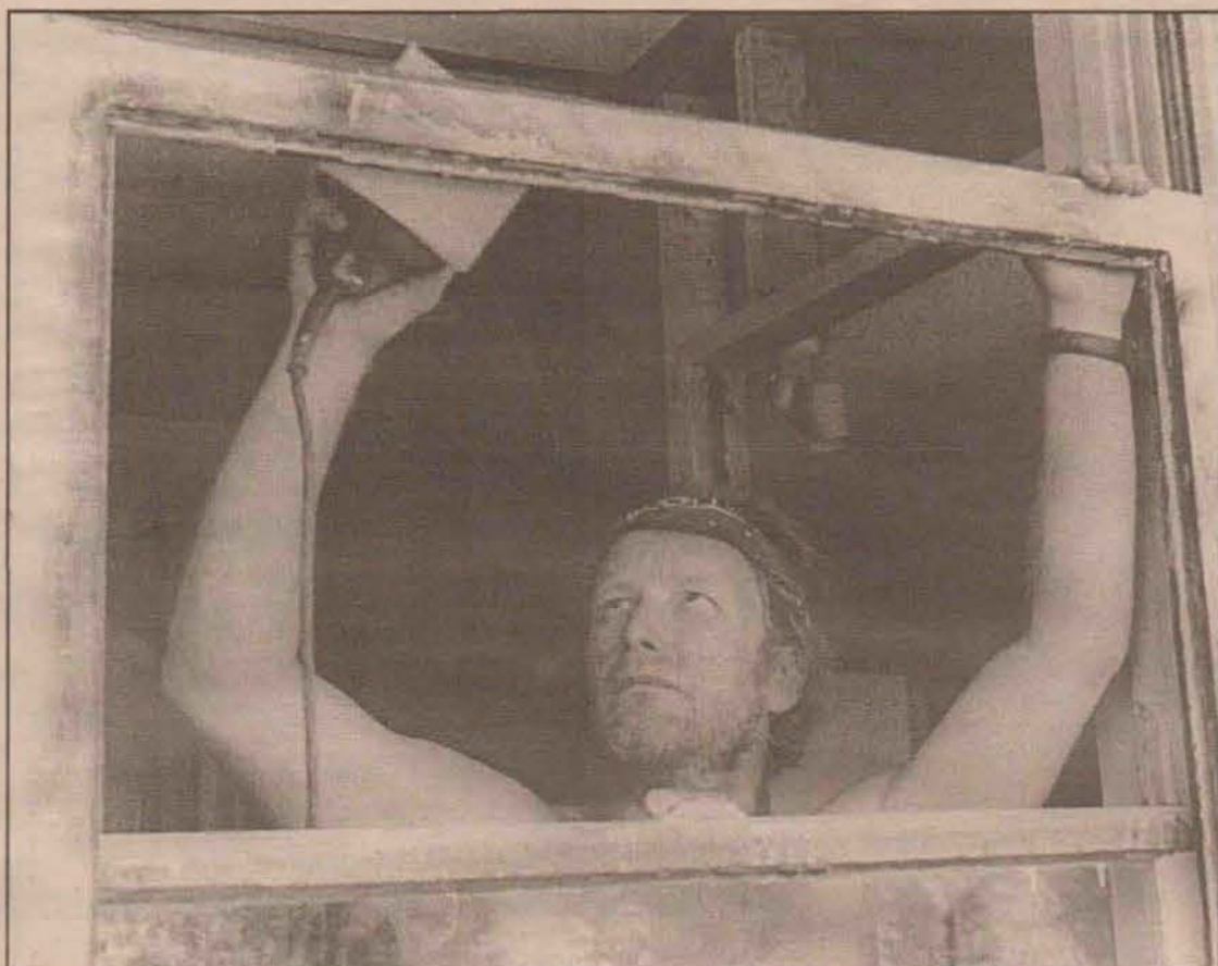
FRAMED: Contractor Bob Jankura sands old paint off second floor windows of the Core Inn. Renovations are under way to create a
