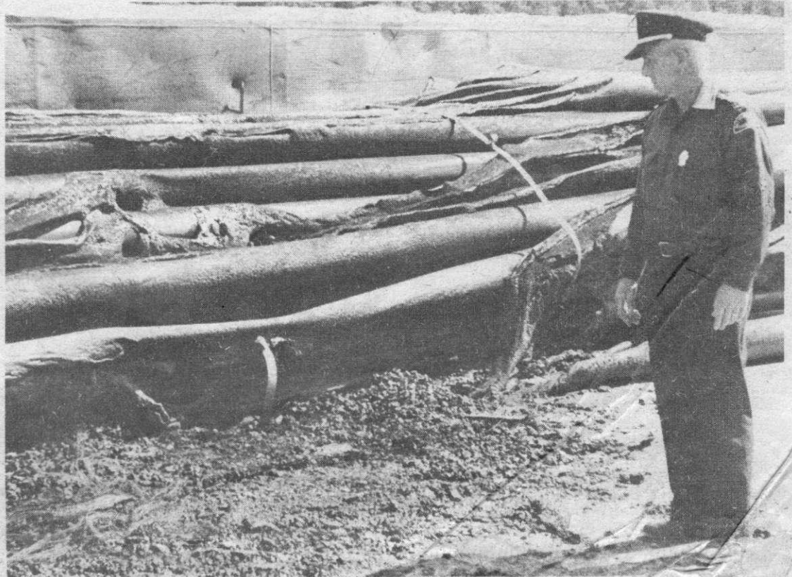
Fire chief Bob Leask and melted plastic outfall pipe. This was one of five places in which fire was started.
