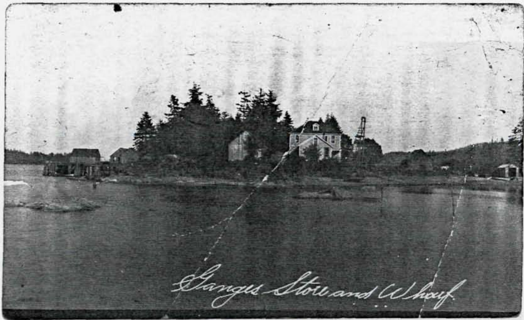
Ganges Store and Wharf Early 1900's
